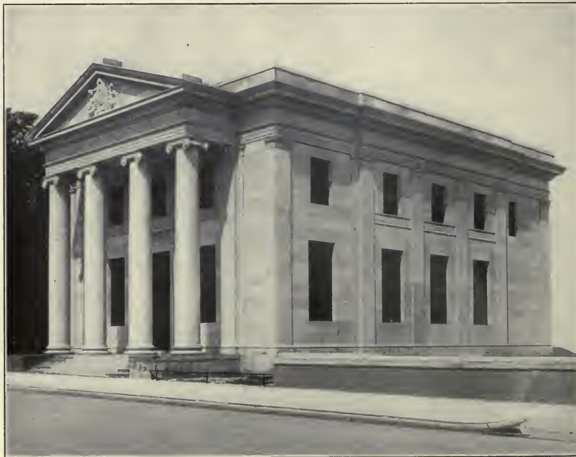
BANK BUILDING ERECTED BY ANGLINS LIMITED.
